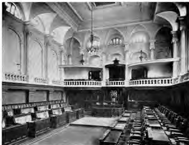
Interior of the chamber of the Raadsaal. The louvres for air-conditioning are high up on the left hand wall.
