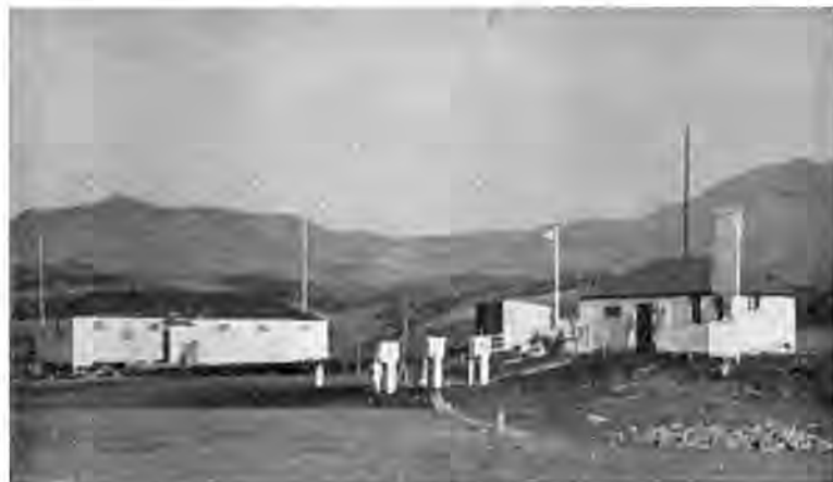
The main buildings on Marion Island, with the Governor's house on the left. The meteorological office is on the right, the radio station masts in the background with the power station in the centre. The Stephenson's screens for recording rainfall, sunshine and temperature are in the middle foreground.
