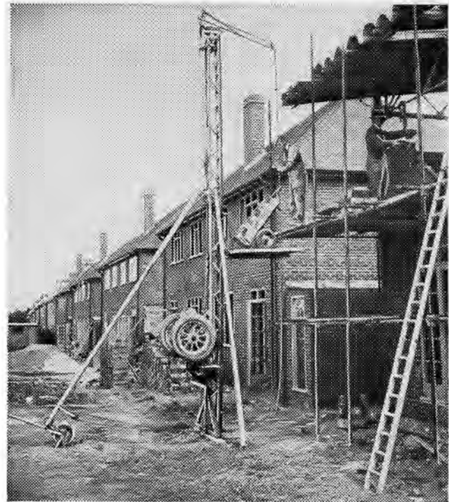
British portable builders' hoist invented by an ex-bricklayer.
