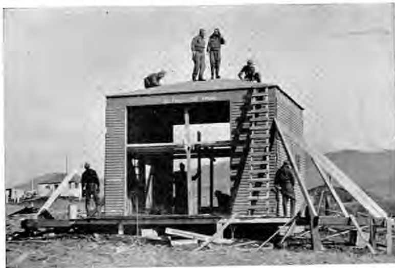
The Radio Sonde Hut under construction.
