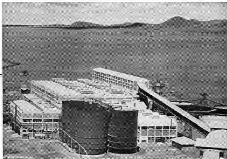
REDUCTION PLANT, LIBANON GOLD MINE
