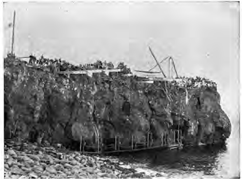
The retractable landing stage and two cranes on the summit of Gunner's Point.
