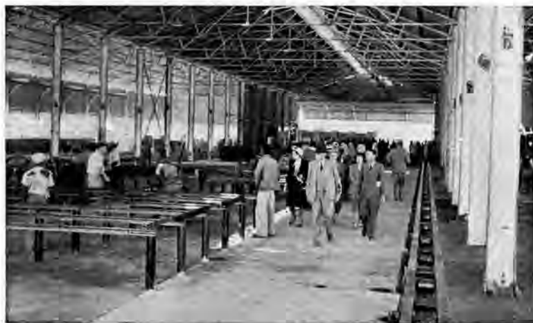
Interior view of the Que-Que tube-works.
