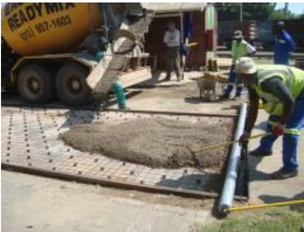
Photo 7 - Casting of concrete
