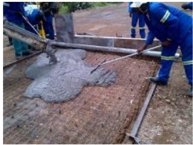
Photo 16 - Casting of concrete
