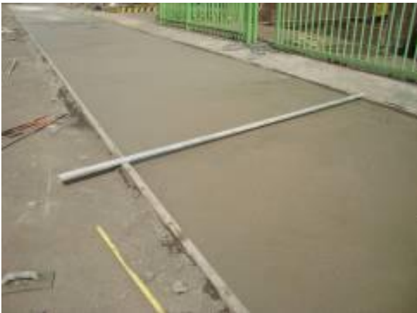
Photo 5 - Preparation of base
