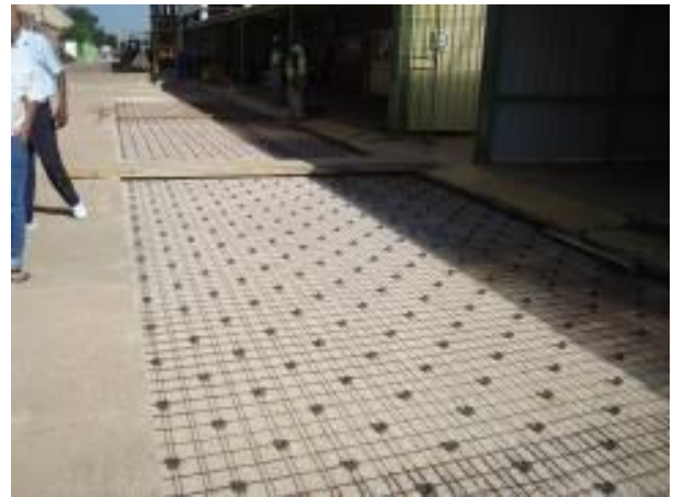
Photo 6 - Preparation of reinforcing
