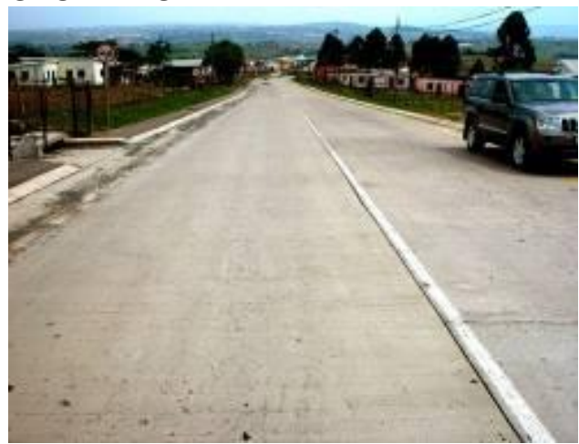
Photo 4 - View of CSIR test section at Soshanguve
