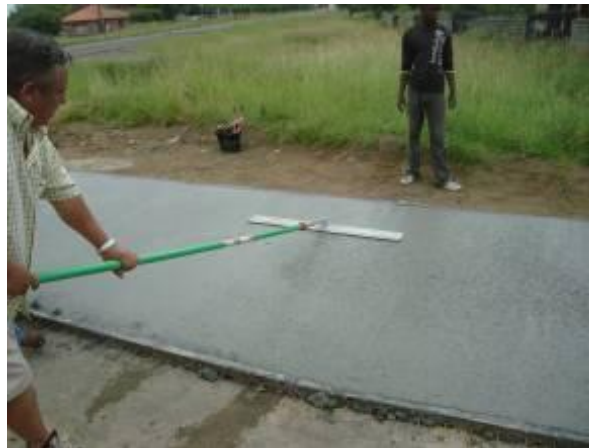
Photo 14 - Floating of concrete with bull float
