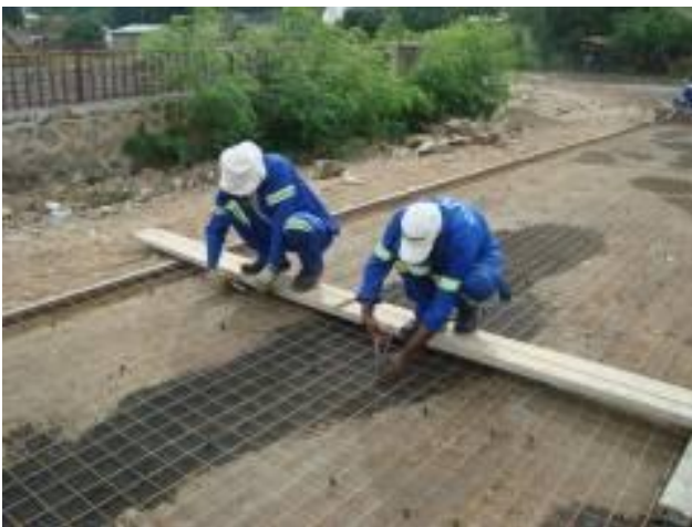
Photo 15 - Preparation of reinforcing
