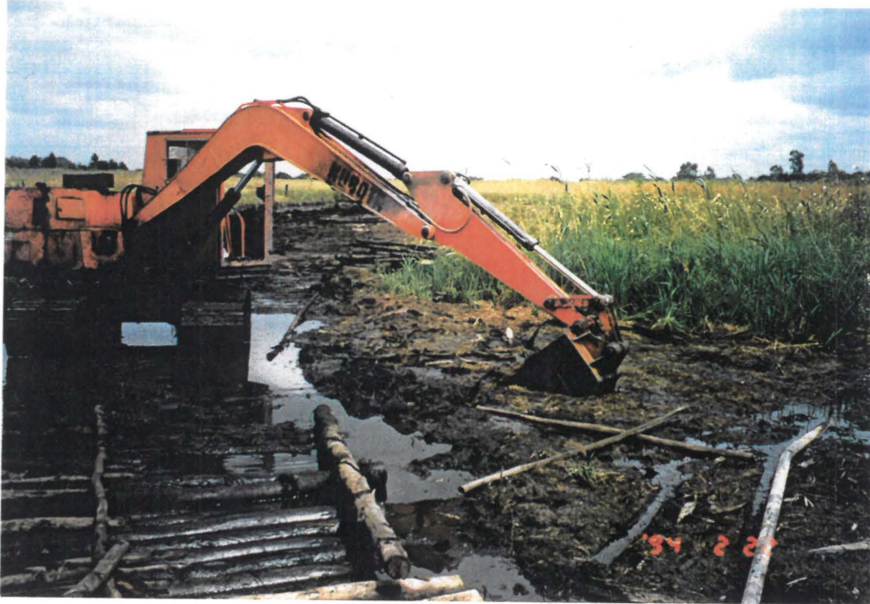
Figure 12 Mechanical digger excavating Potchefstroom reed-sedge peat.
