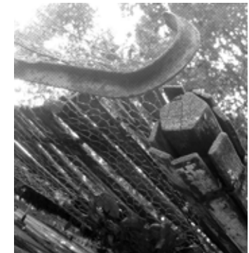
Fig_107: Roof detail with timber louvers.
