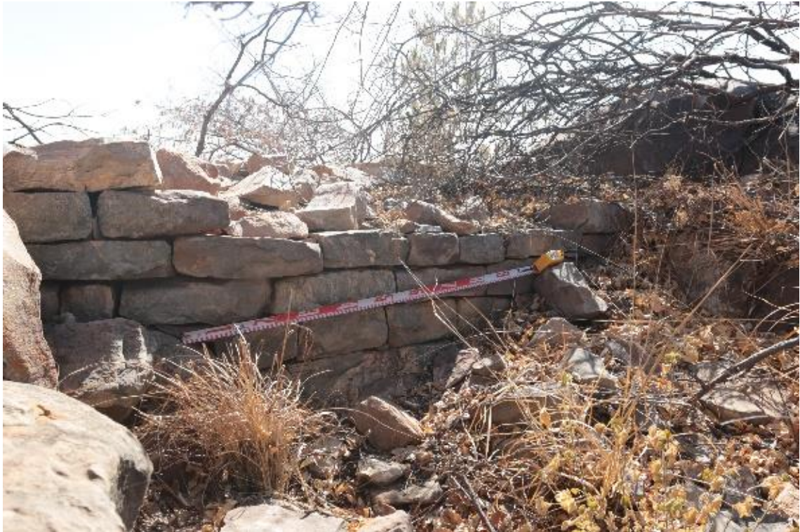
Figure 6-141: step at entrance to high status area
