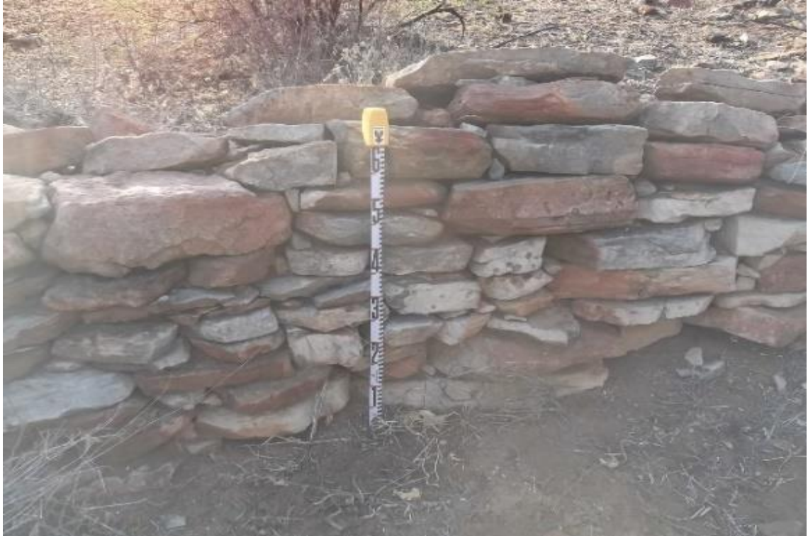
Figure 6-103: formal walling on the western section of the site
