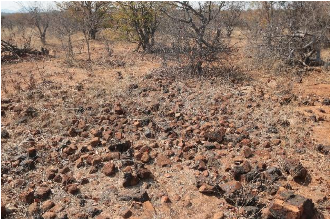
Figure 6-123: collapsed brick structure
