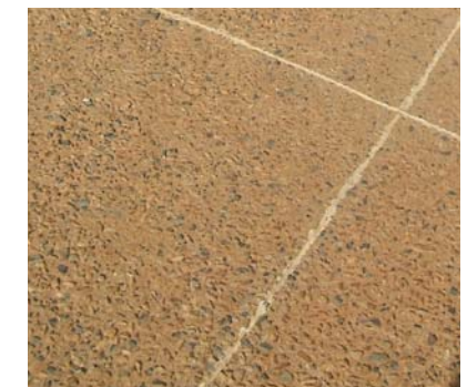
Illus. 9.7: Exposed aggregate concrete (Author, March 2009)
