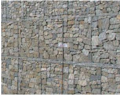
Illus. 9.3: Packed gabions to be used as seating walls ( www.gabionbaskets.co.za )
