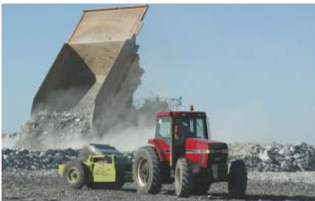
Figure 1. The “square” impact roller on a mine waste tip.
