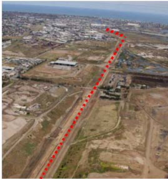
Figure 3. Aerial view of the Port River Expressway (Route: ---).
