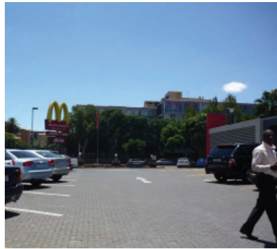
Figure 3.32: Existing single storey building, currently used by McDonalds, to be demolished (Author)
