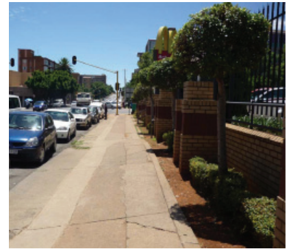
Figure 3.34: Illustrating the dead city sidewalk caused by the un-interactive palisade fence around the site (Author)
