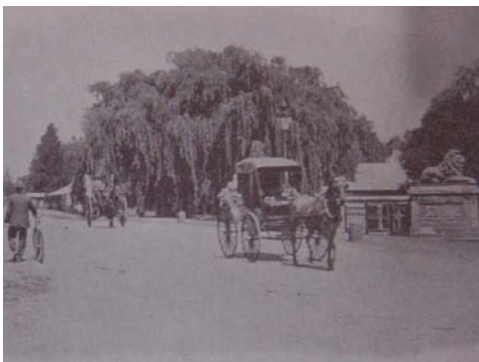
Figure 3.25: A photo taken later of Lion's bridge. The four bronze lions were cast in Scotland by MacFarlane Sun Foundry (Swanepoel, 2007: 10).
