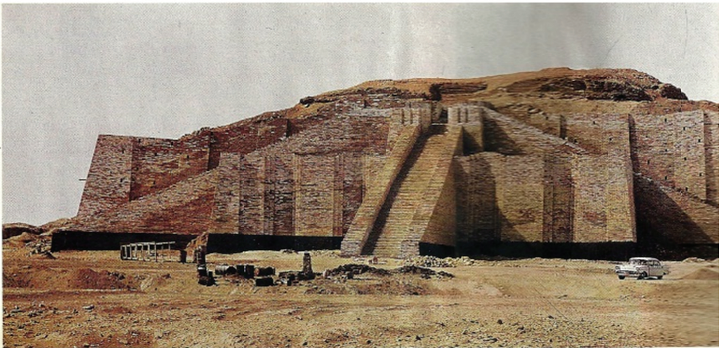
FIGURE 1.9 Ziggurat of Ur. Ca. 2100 B.C. Ur (Muqaiyir, Iraq). A temple to Nanna, the moon god, stood on the top of the ziggurat, which was terraced on three different levels. On the first level was an entranceway approached by two sets of steps on each side and one in the front. The base measured 200 by 150 feet and stood 70 feet high.
