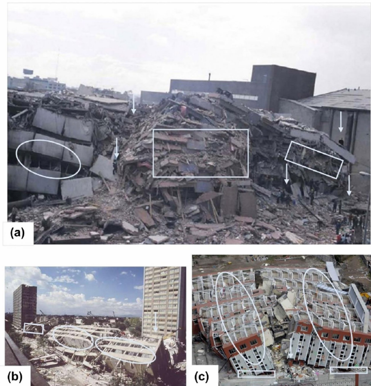
Fig. 2 People trapped in rubble from collapsed buildings due to an earthquake (Reinoso et al. 2018)
