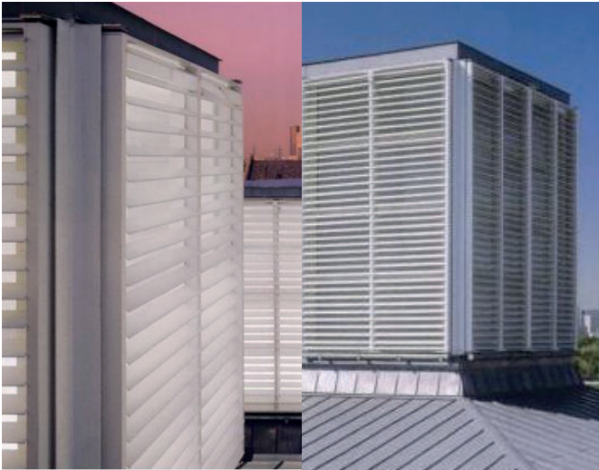
Figure 7.25: Examples of sky lanterns acting as skylights letting light in through glazing located on the sides with incorporated diffusers.
