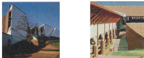
Figure 7.8: Photos showing the clay sunscreen and the terracotta roof tiles laid on asbestos
