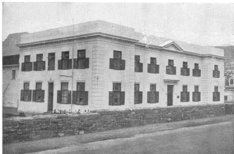
ADMINISTRATIVE AND LABORATORY BLOCK.
