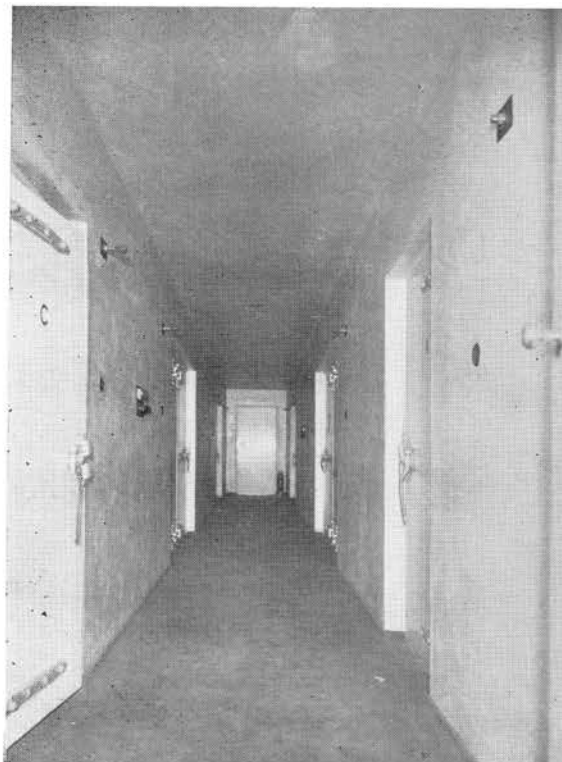
COLD STORAGE CHAMBERS LEADING OFF ONE OF THE CORRIDORS.
