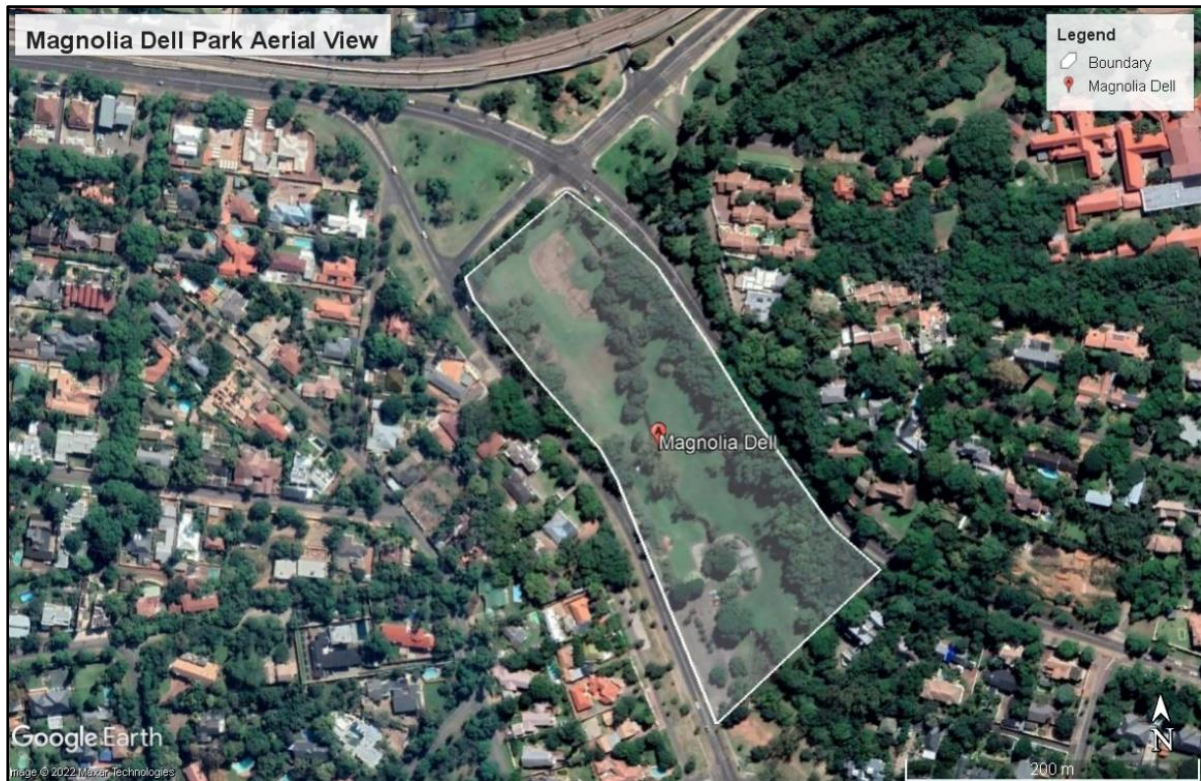
Figure 1.6 Magnolia Dell Park Aerial View
