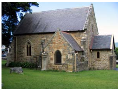
3.21. The original Anglican Church in Main Road which was the first church to be built in Knysna (1849-1855) (Howard 2005)
