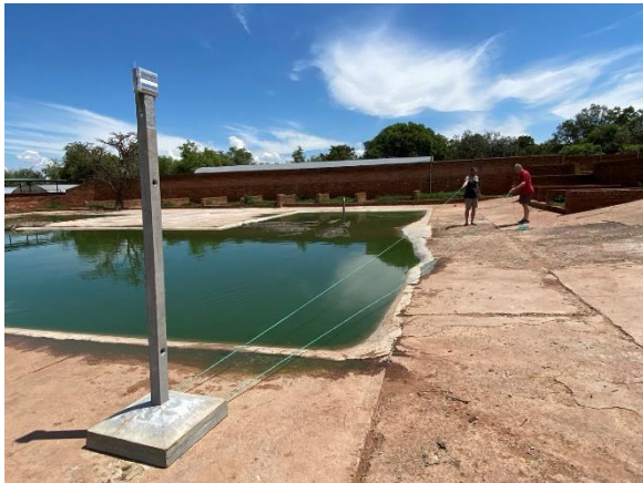
Figure A15. The steel pole in a concrete base design, with the LHT65 logger box secured up top, before being pulled into the waterbody.
