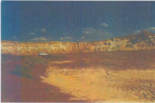
Fig. E.1 - Study site A. Partially reclaimed. Dam height approximately 15-20 metres.
