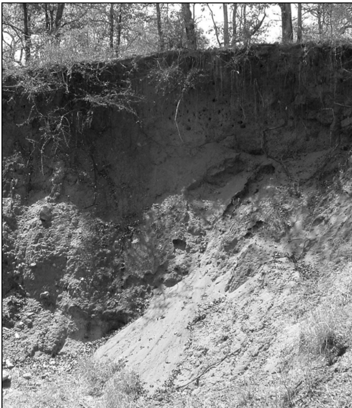
Figure 38: Sidewall of donga that cuts through BS04.
