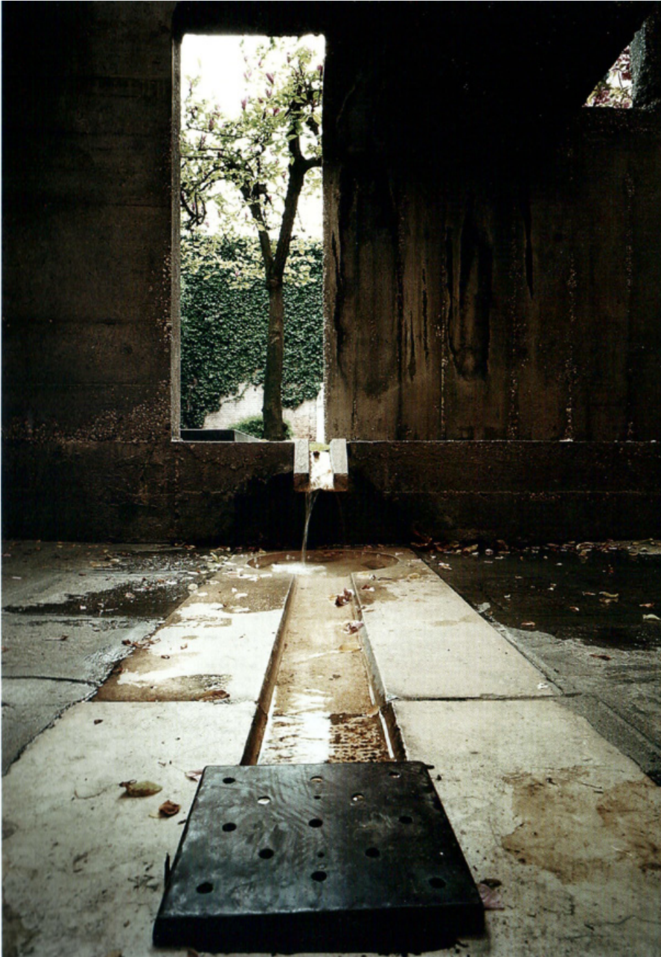
Fig. 5.24 Photograph showing dialogue between the built fabric and nature. Photograph by Alessandra Chemollo (2003).
