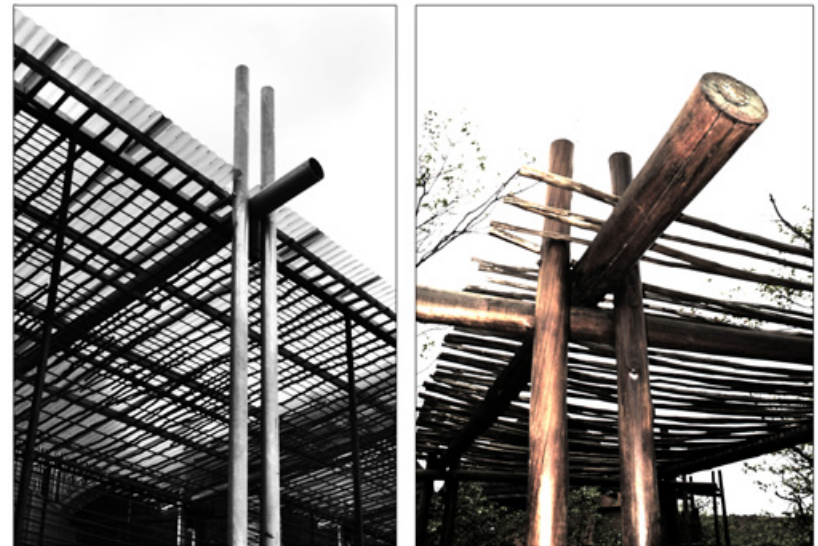
Fig. 5.06 Photographic comparison between traditional timber gum pole construction and the steel construction interpretation at the interpretation centre. Photographs by author.
