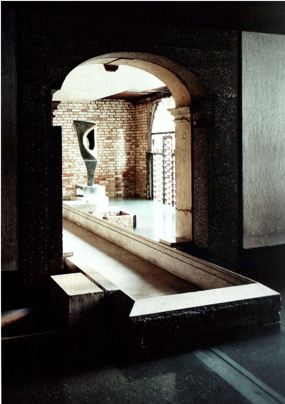
Fig. 5.21 Photograph showing the elevated walkway separated from the flooding process. Photograph by Chemollo, A (2003).
