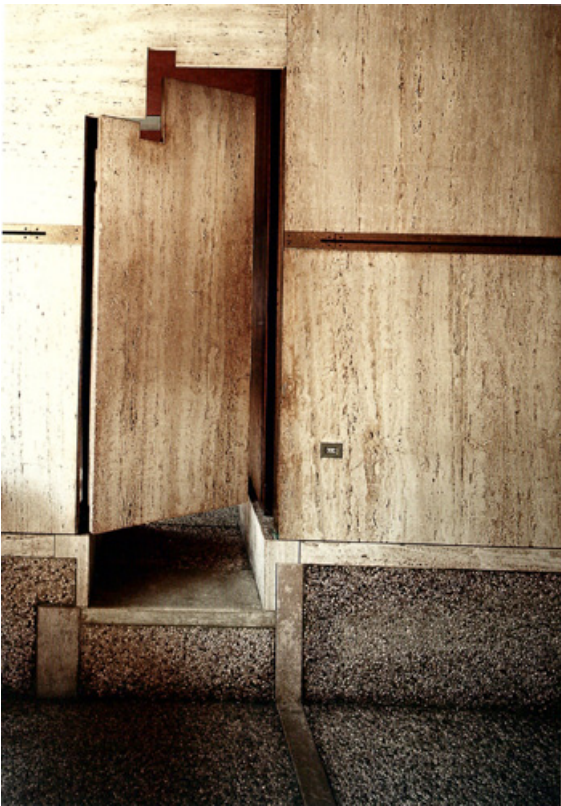
Fig. 5.19 Photograph showing the flood line represented on the wall of the exhibition room. Photograph by Chemollo, A (2003).
