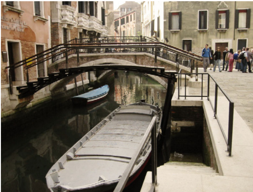
Fig. 5.17 Photograph of bridge spanning over the existing canal to articulate the entrance to the palace. Image from en.wikipedia.org (Accessed 15 August 2012).
