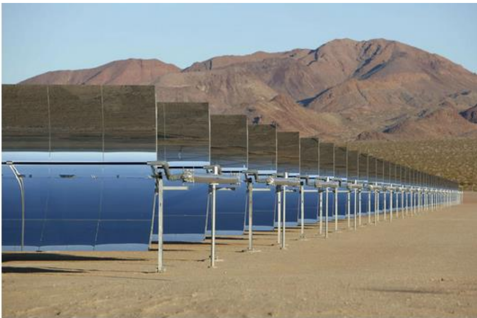
Figure 1-4: Solar-power plant with a concentrated array [10].
