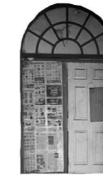
TIMBER FRAMING REUSED SIMILARLY Available from the 'white house'
