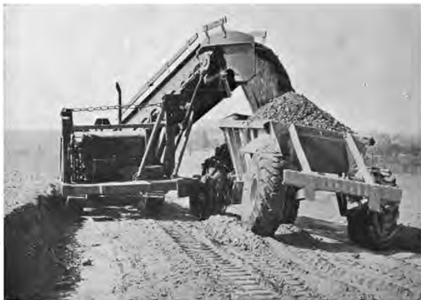
The Euclid Loader and Bottom Dump Wagon in operation, shewing the depth of cut.
