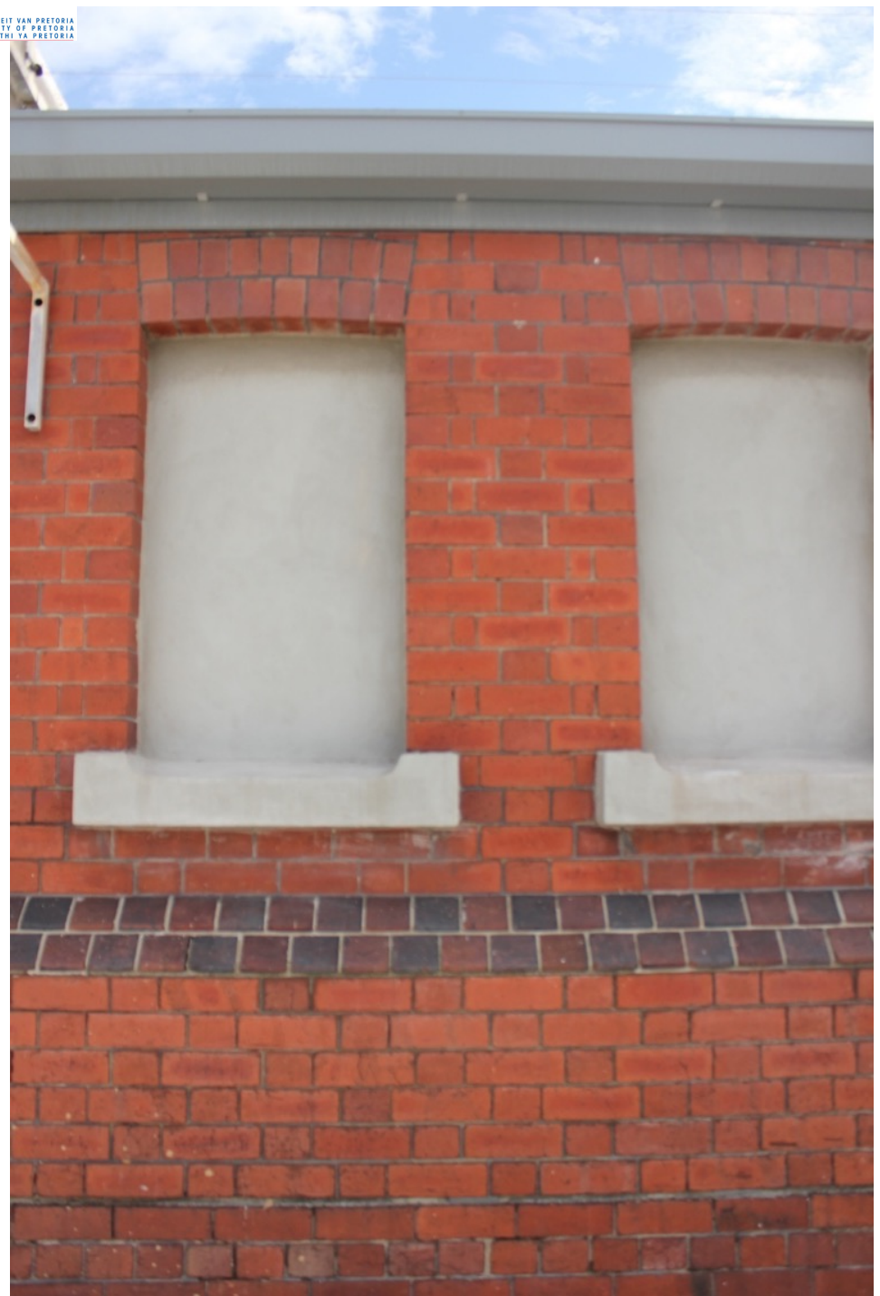
Figure 226: Photograph of brick detailing, southern facade: (Author 2021)
