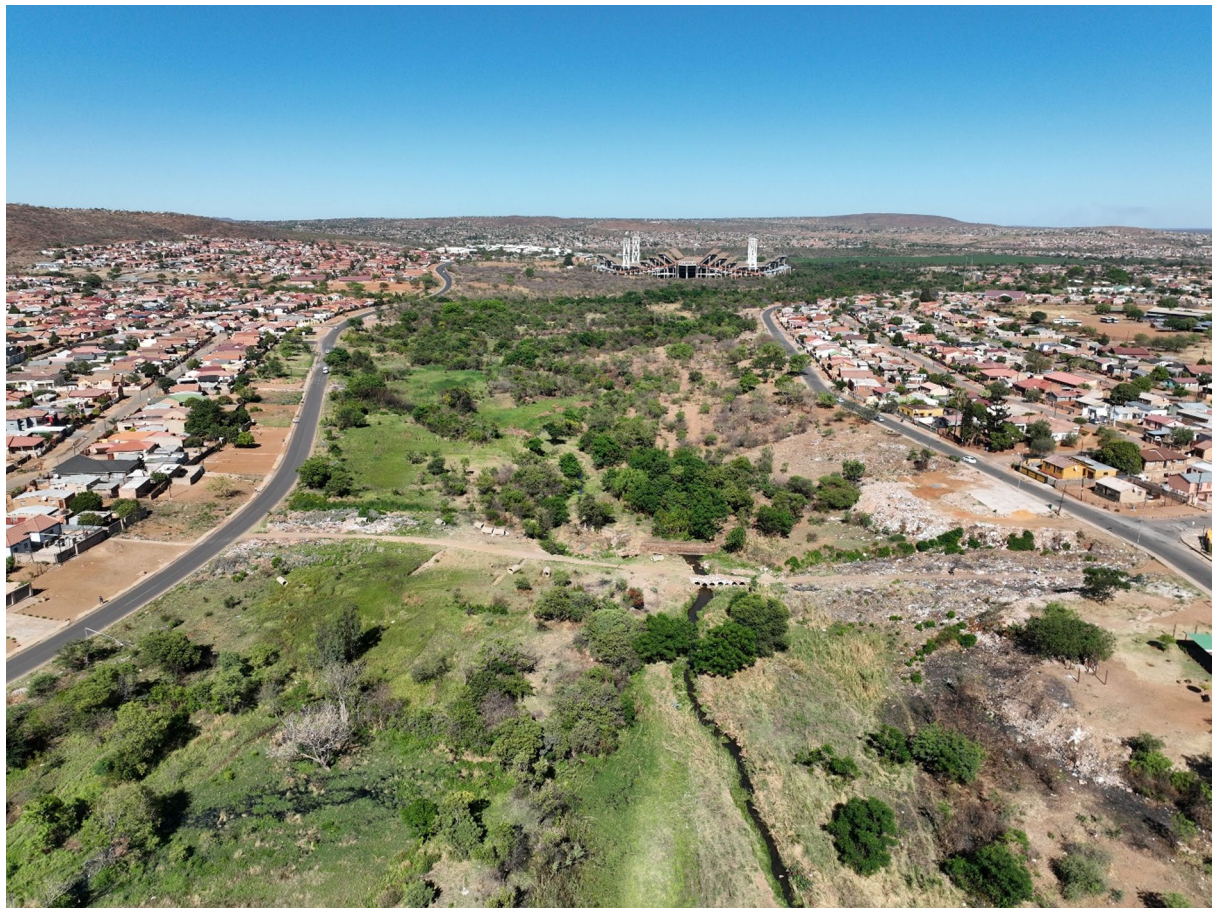
Fig. 3. Bird's eye view of the study site looking west with the north-south river crossing in the centre and the Odi athletics stadium and Magaliesberg mountain range in the background. Dumping of domestic waste and building rubble can be observed along the green space edges and the river crossing (Photo credit: S Küssel).
