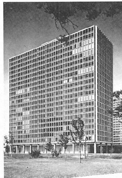
Figure 6 Detroit apartments (Alexander 2002:329)
