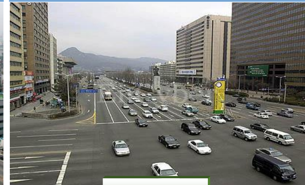
Pedestrian Crossing Re-establishment
