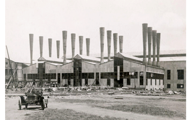
Fig 75 Rosherville Power Station (Eskom, n.d)
