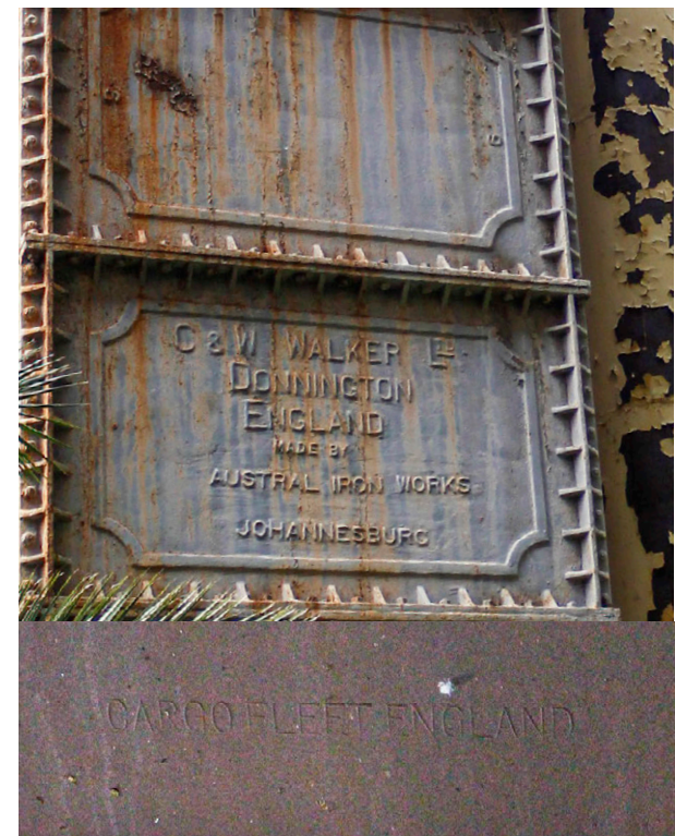
Fig 44 Engineers signature on steel
