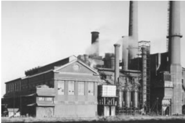
Fig 76 Congella Power Station (Eskom, n.d) energy production method Coal fired
