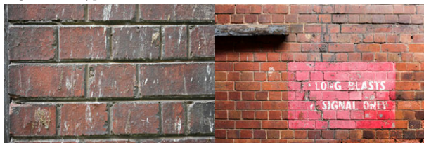
Fig 40 English bond brickwork
