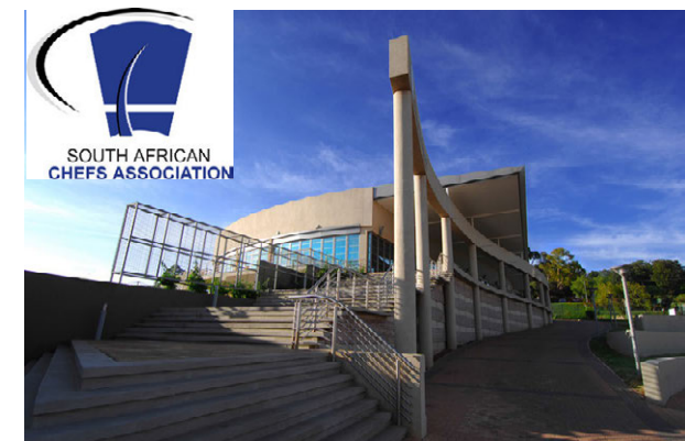
Fig 111 The Kerzner Building (University of Johannesburg, 2017)
