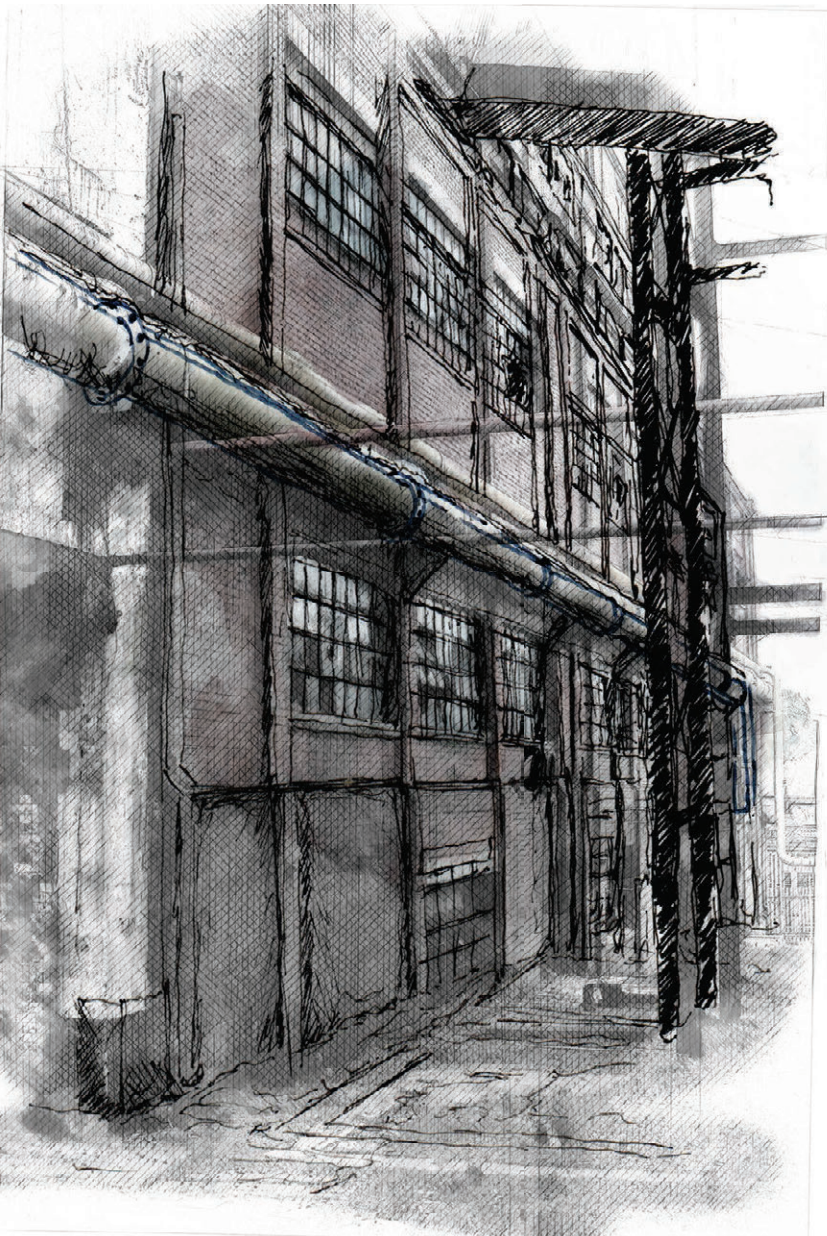
Fig 130 View down southern facade
