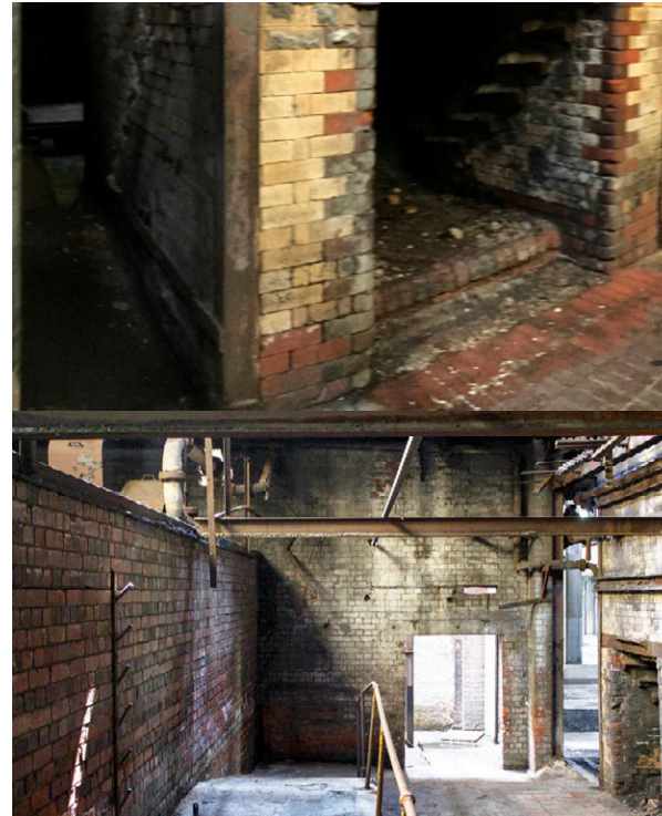
Fig 187 Boiler house & unique detailing
