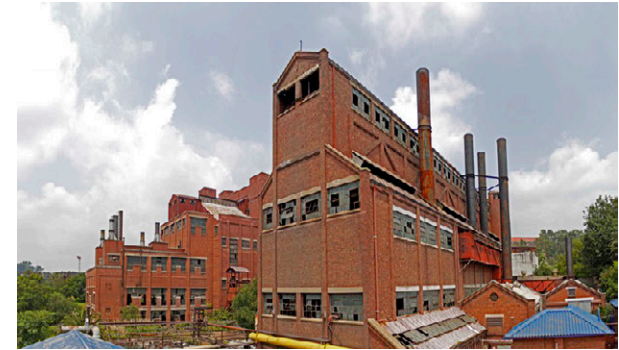
Fig 6 The first Retort, the Johannesburg Gas Works
