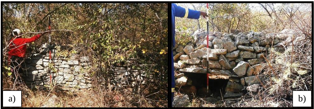
Plate 5.17: a). A section with PQ walling on Arupanga enclosure located at the western foot of the hill, b). Lintelled opening of Arupanga enclosure showing R-style walling technique
