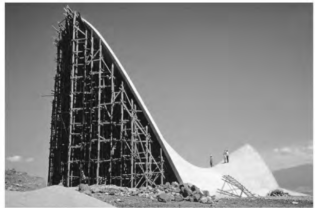
Figure 23: Material-intensive formwork of a concrete shell by Candela (Pereira 2018)
