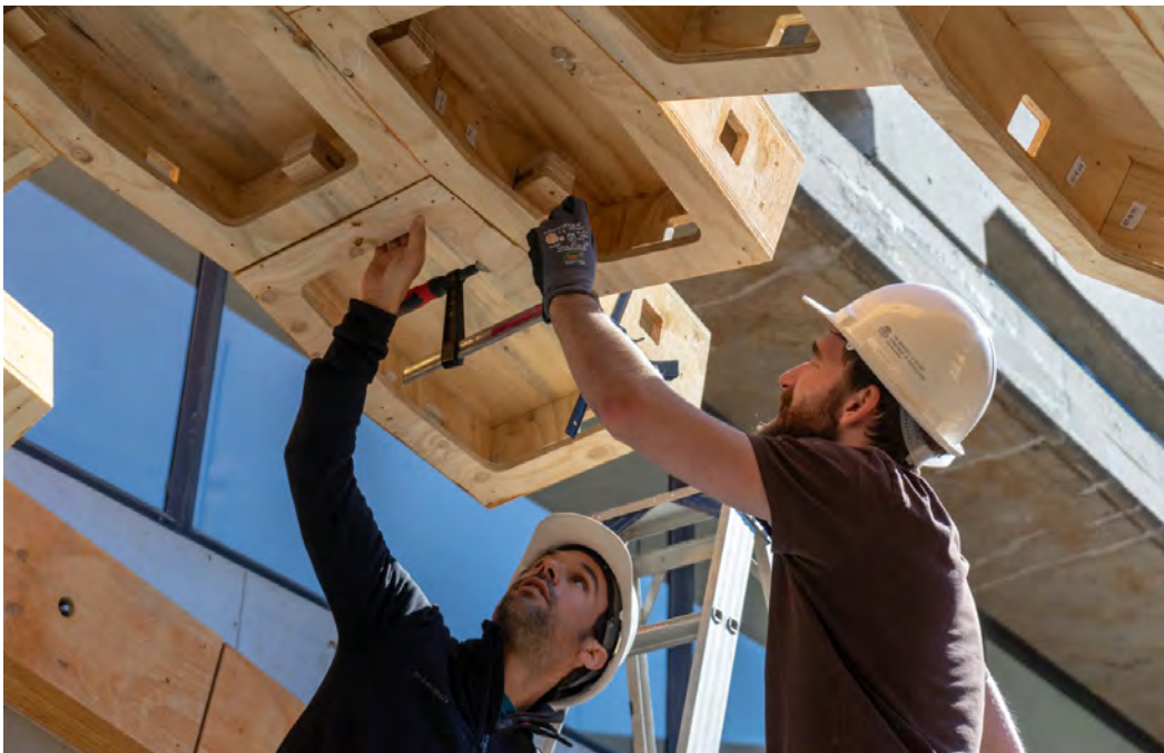
Figure 33: Assembly process for HexBox Canopy (Pintos 2019)
