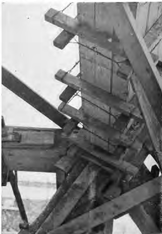
INTERSECTION OF HORIZONTAL, CIRCUMFERENTIAL AND DIAGONAL BRACING, IN TRESTLE CONSTRUCTION.
