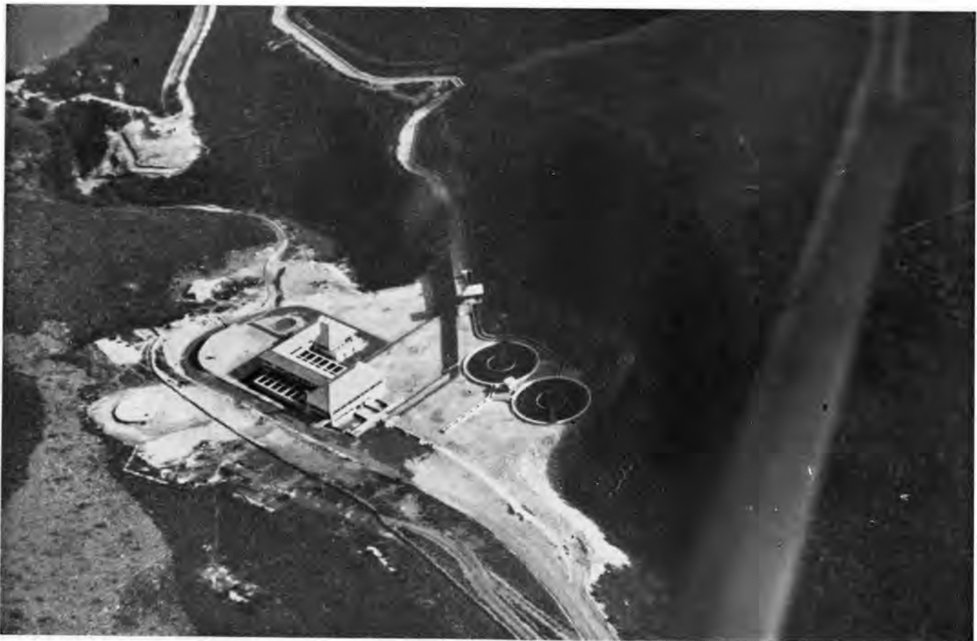
VIEW SHOWING CANAL TO PURIFICATION WORKS.
