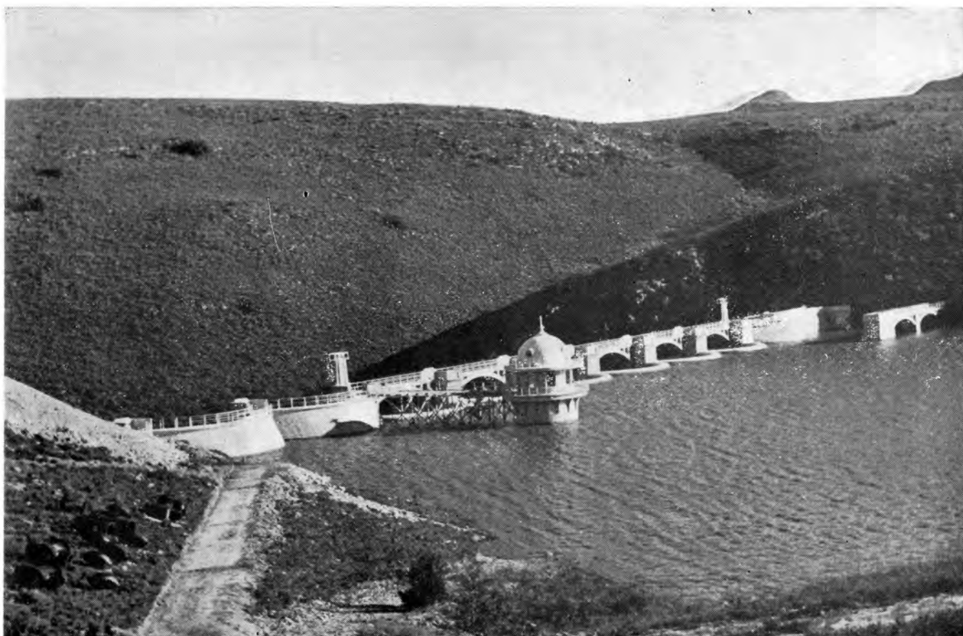
GENERAL VIEW FROM THE UPSTREAM SIDE OF DAM PORT ELIZABETH.
