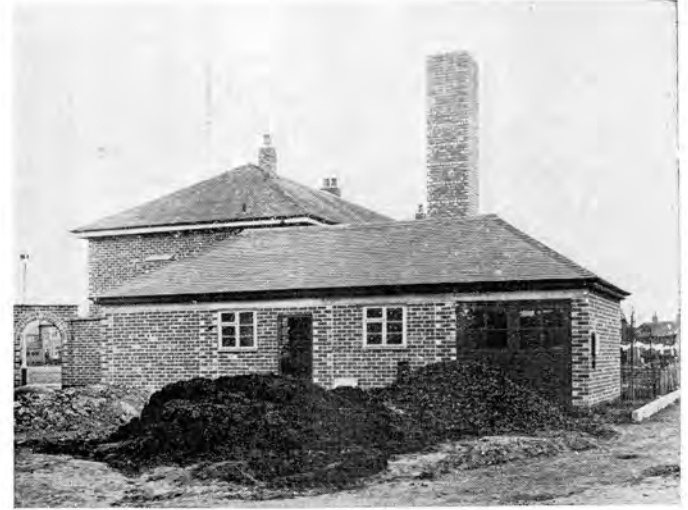
CENTRAL BOILER HOUSE AND PUMPING STATION.
