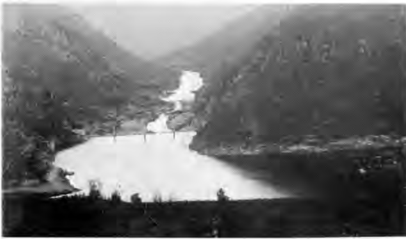
KROMME RIVER GAUGING WEIR.
