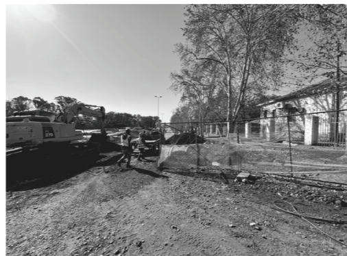
Affected main route to the school, unsafe cycling conditions for school kids
