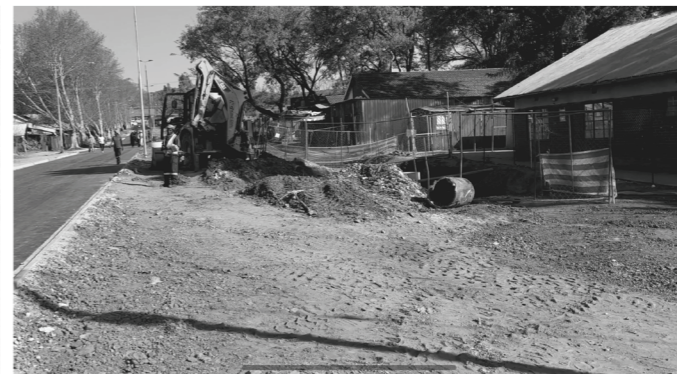
Demolished front yard for road extension
