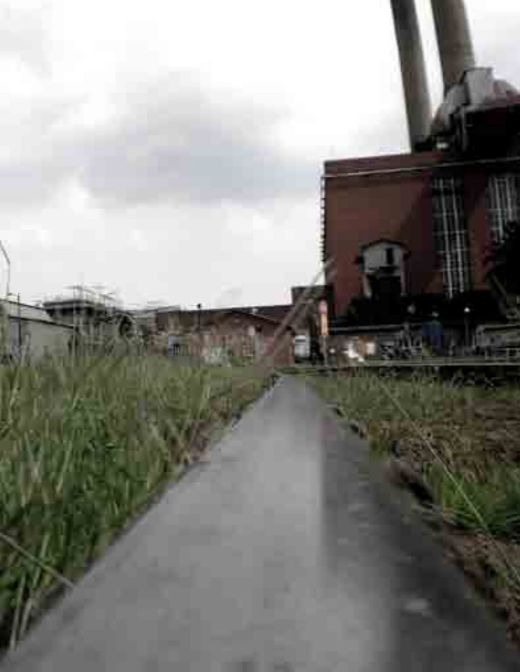
fig. 22_ Existing railway track on site, power station in background
