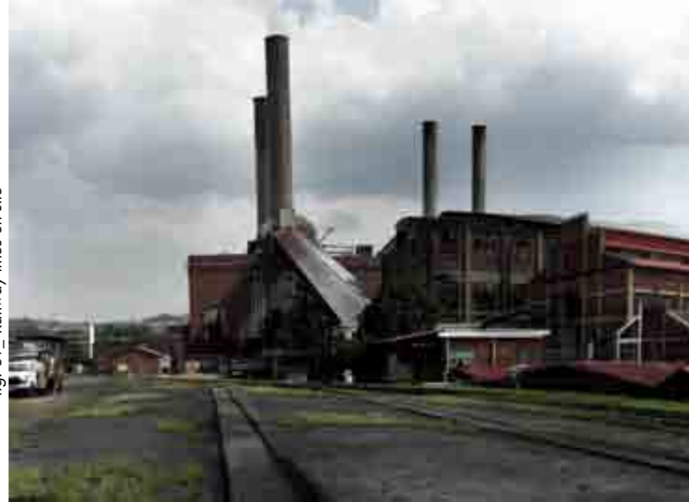
fig. 39_ Railway lines on site
