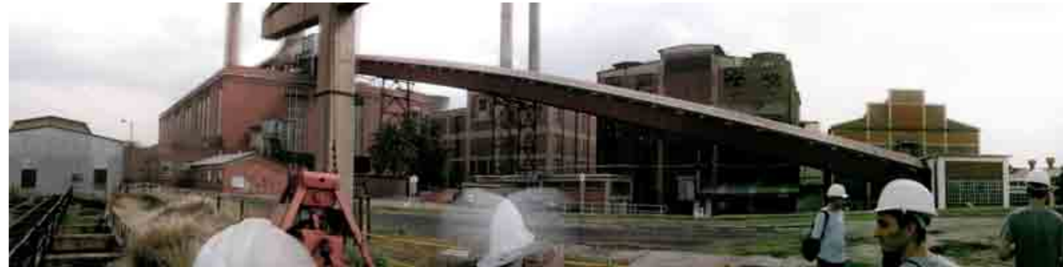
fig. 41_ Photograph of structures on site
