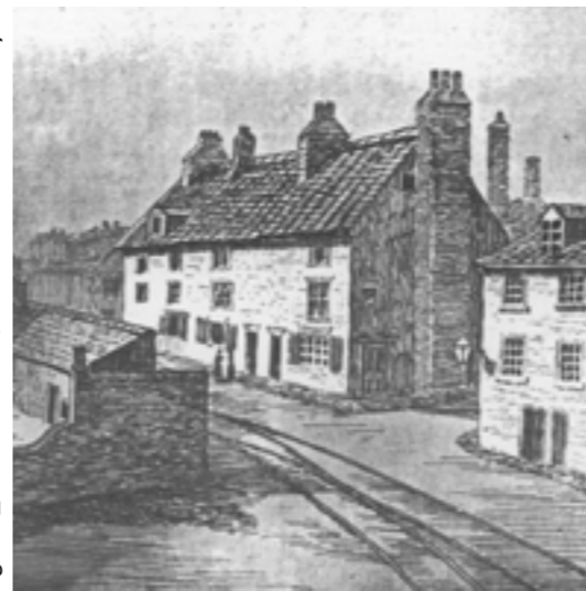
fig. 13_ The Fleese Inn, at one end of the railway line, 1823
