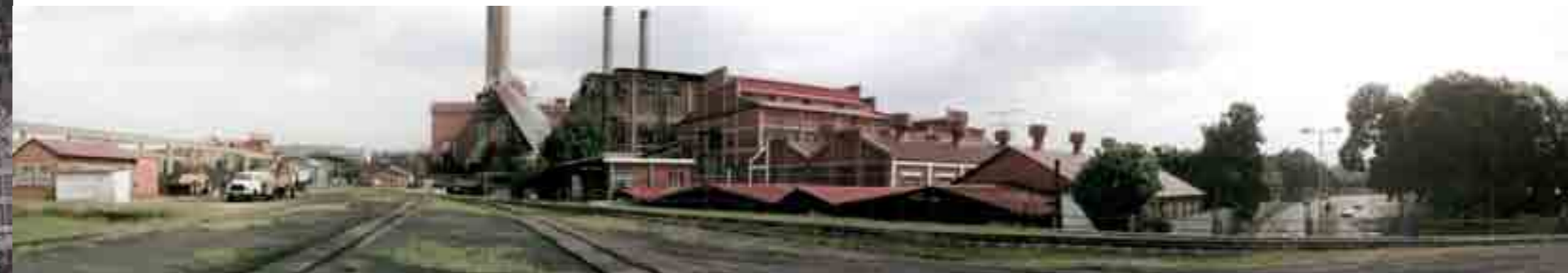
fig. 37_ Panoramic of buildings on site [earliest right - latest left]
