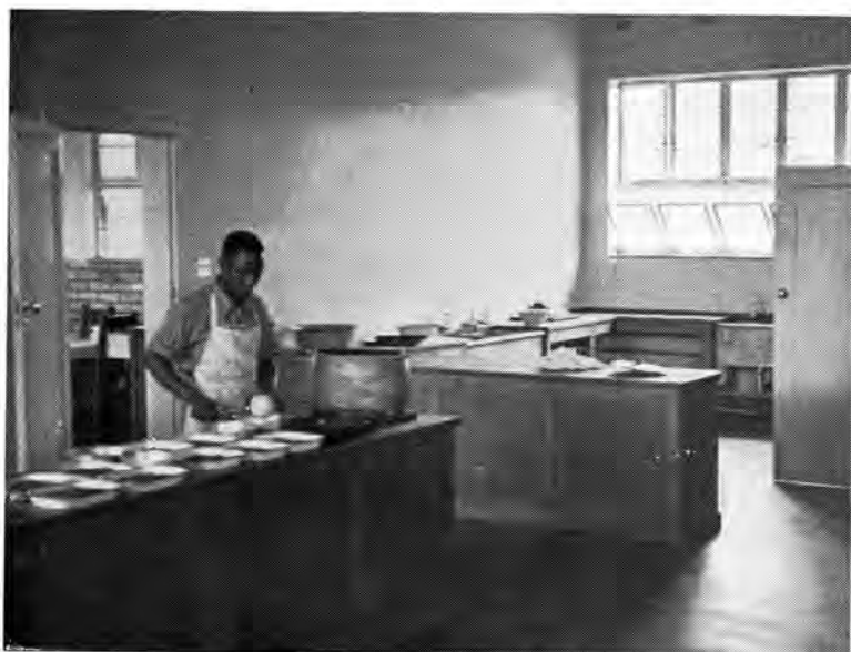
Preparation end of kitchen; cooking is by anthracite-burning heat insulated stoves.
