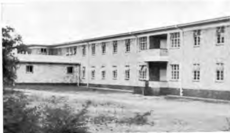
North aspect of girls' dormitory block showing staff wing projecting.
