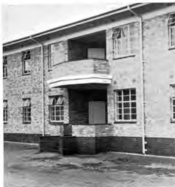
Porch and Verandah to Staff Rooms.
