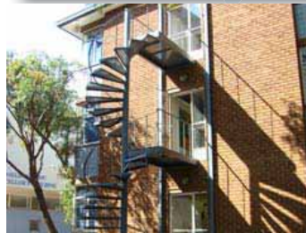
Spiral staircase at Marketing building
