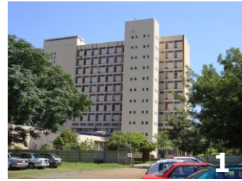
Fig 26. Neighbouring building on northern side of the site
