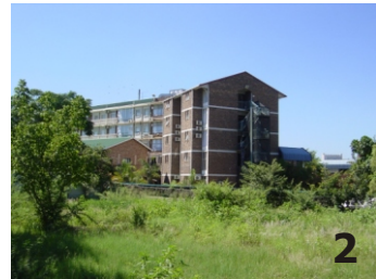
Fig 27. Neighbouring building on south-eastern side of the site
