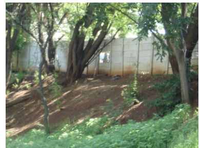
Fig 16. View of wall from Apies River
