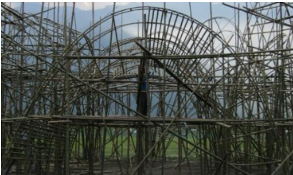
Bamboo sheathing is installed for vaults with primary structure rigid and complete steel rings for woodwork decking is welded to steel pipes.
