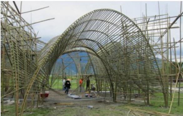
Scaffolding is removed from each completed vault and wood decking installed.
