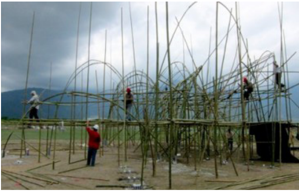
Primary structure of vaults are erected, with scaffolding as needed.
