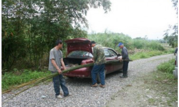
Bamboo is freshly cut from nearby forests and transported to site in small increments
