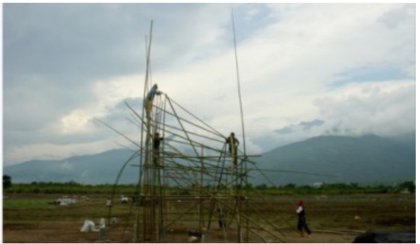
Primary arcs and main spanning are erected, with scaffolding for support as needed.
