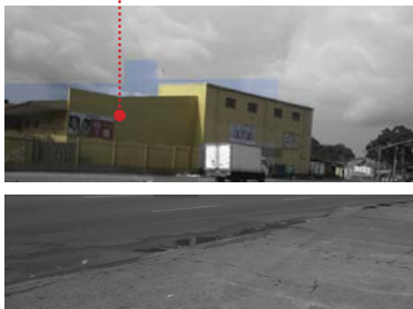
Fig 7.113 Photo of industrial building (Author, 2014).
