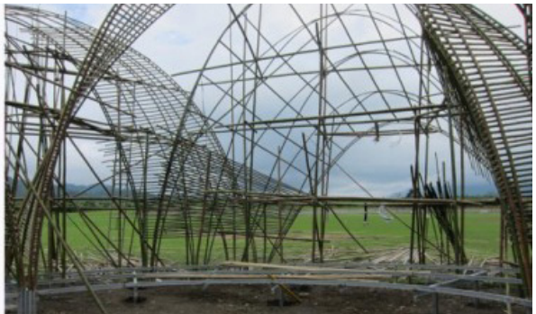
Bamboo sheathing is installed for vaults with primary structure rigid and complete steel rings for woodwork decking is welded to steel pipes.
