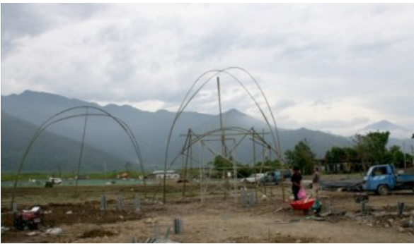
Primary arcs and main spanning are erected, with scaffolding for support as needed.
