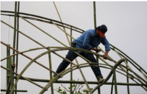
Bracing arcs are erected, weaving in between scaffolding and vault.
