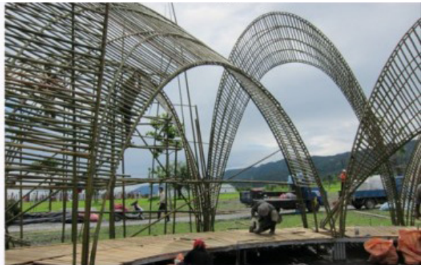
Bamboo sheathing is installed for vaults with primary structure rigid and complete steel rings for woodwork decking is welded to steel pipes.
