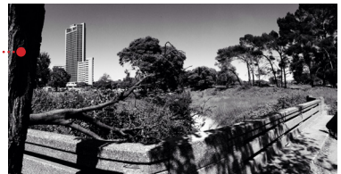
Fig 4.29 Bridge over Bloed Street (Author, 2014)
