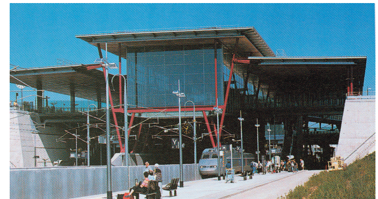
FIG 020 Section and photograph illustrating the central glass box floating over the platforms and tracks
