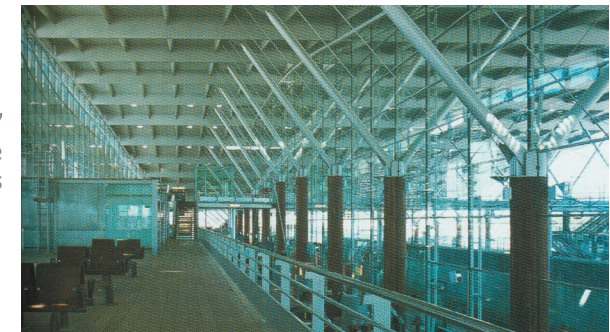
FIG 027 Mezzanine levels and bridges offer an overlook on the Aix-en-Provence station activities
