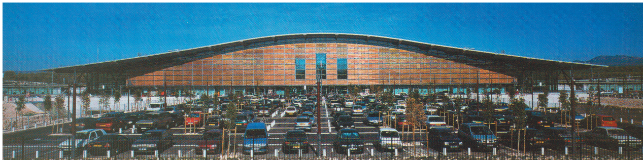
FIG 025 Aix-en-Provence's curving facade indicates the station entrance
