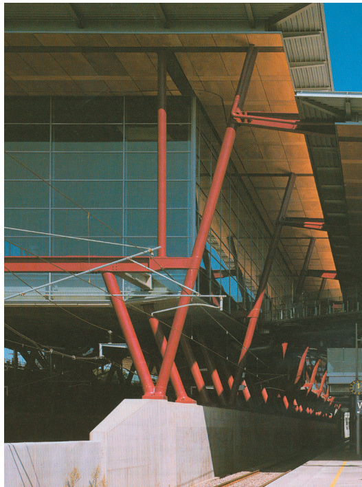
FIG 022 Duality - robust concrete platforms in contrast with the glass and steel station structure
