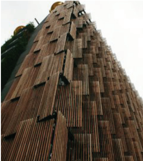
Figure 5.20: Timber shutters for units (Online)
