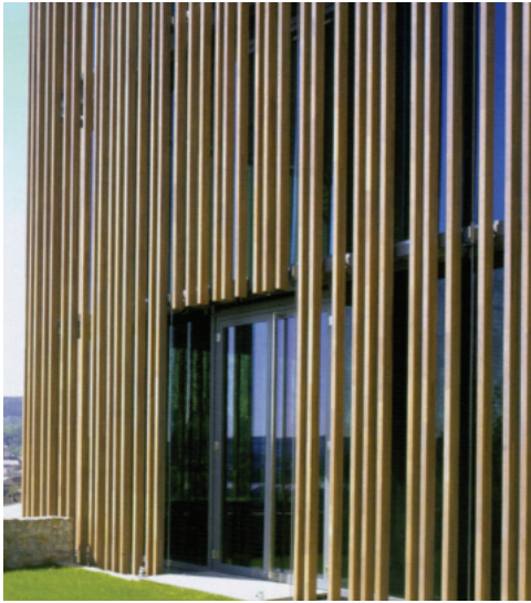
Figure 5.19: Shelter entrance – timber screen, transitional layers (Messedat, 2007: 223)
