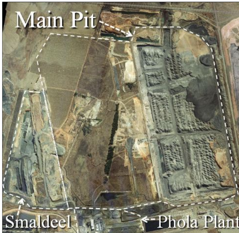
Figure 1.2: Klipspruit Colliery Sections
