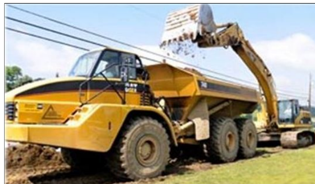
Figure 3.5: Topsoil Truck and Shovel Operation
