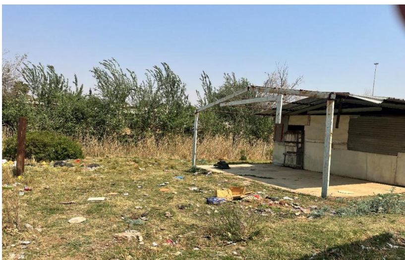
Photo 2 (P4:2) shows unmaintained grass and overgrown trees.
