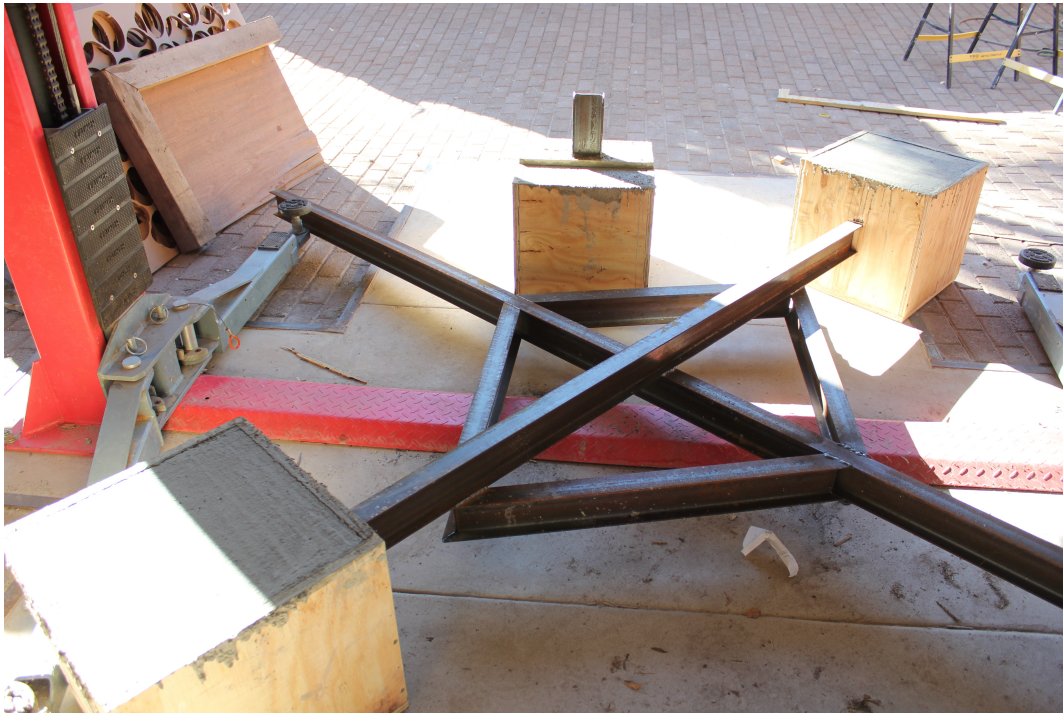
Figure 110: Cast concrete fuselage blocks
