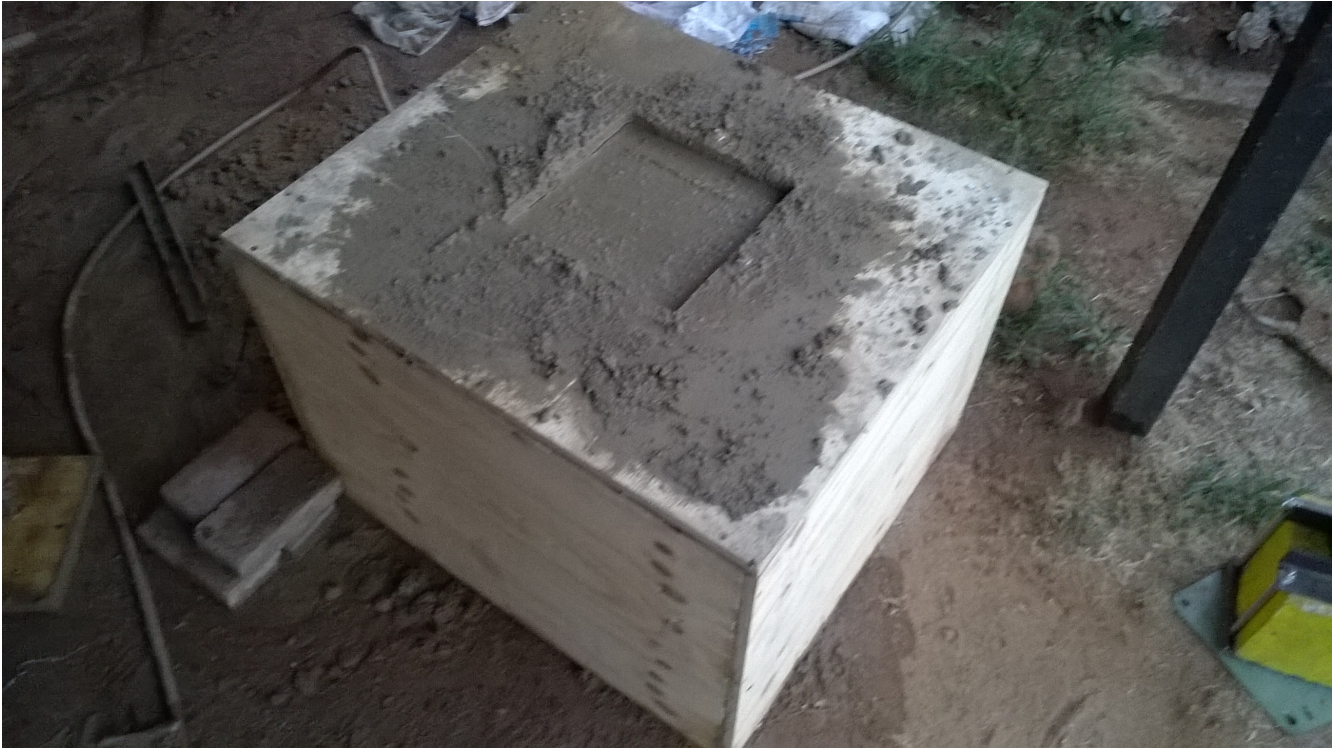
Figure 57: Dummy fuselage cast concrete
