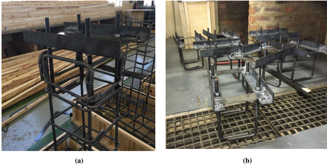
Figure 3-18 Holding down bolts and template
