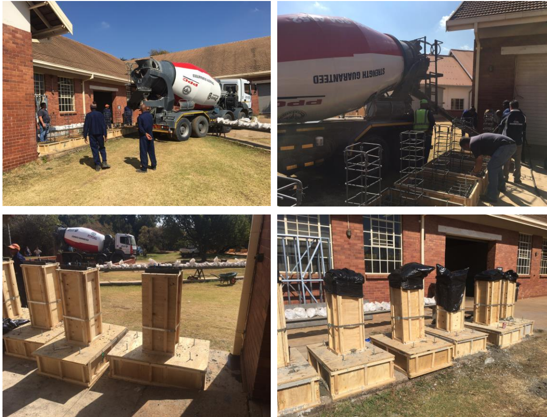
Figure 3-19 Concrete casting of the reinforced concrete footings
