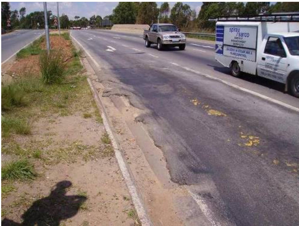
Figure 1 Typical permanent deformation development at an intersection
