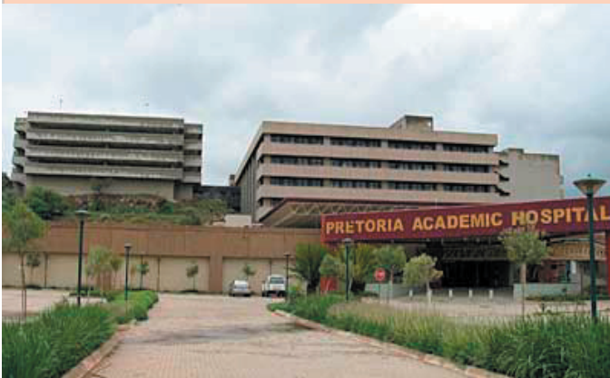
Figure 2.6: New Pretoria Academic Hospital Architects: Leap/MMA
