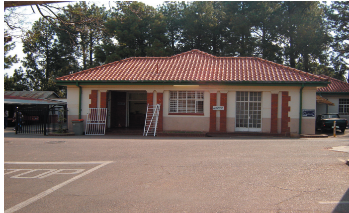
Figure 2.19: Existing hospital mortuary, heritage building
