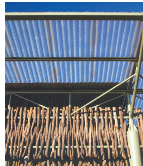
Figure 4.8 Sun-screen detail
