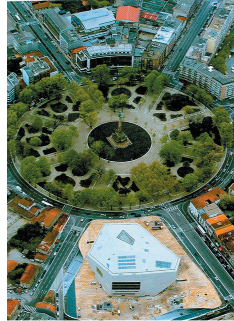
Figure 4.11: Bird's eye view showing Casa Da Musica next to Rotunda Boavista
