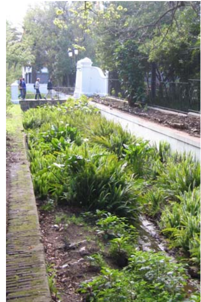
5.26. Vegetated channel (Howard 2005)
