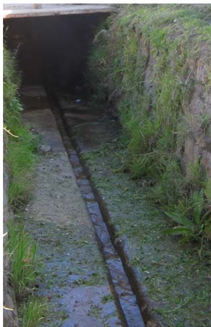
5.16. A concrete channel which has no ecological value (Howard 2005)
