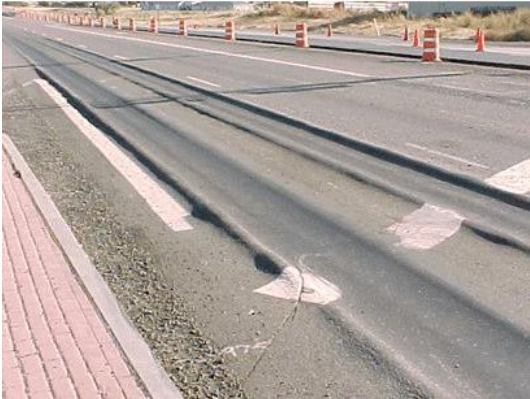
Figure 2-6: Permanent deformation (rutting)
