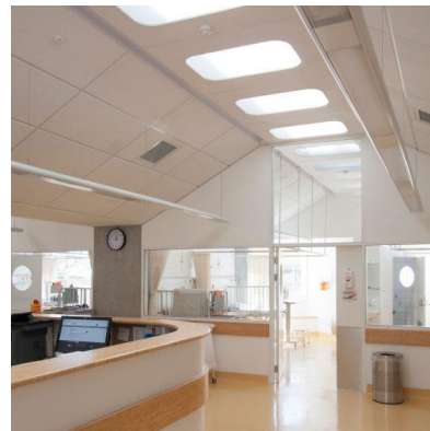
Figure 83: The timber provides warm tones at Vredenburg Hospital, completed 2017 (Wolff Architects, 2024:online)
