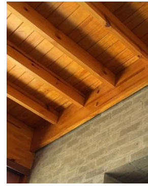
Figure 77: Underside of SA pine roof structure (Wolff Architects, 2024:online)
