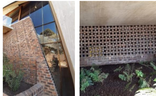
Figure 33: Brickwork at House Fitzgerald. (Author, 2021)
