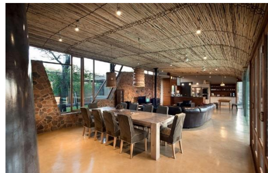
Figure 36: House Mouton, 2014 (Earthworld Architects, 2024: online). The stone walls, timber lathes and concrete floors all retain their natural appearance.
