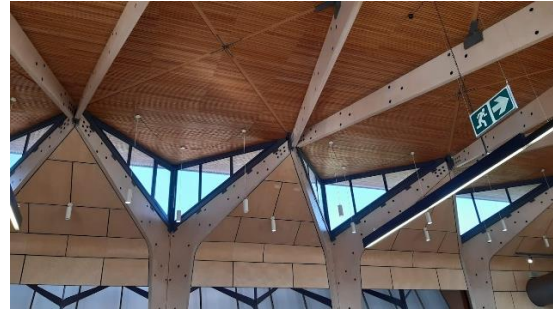
Figure 40: Dining hall at Future Africa Campus, completed 2018 (Author, 2023)
