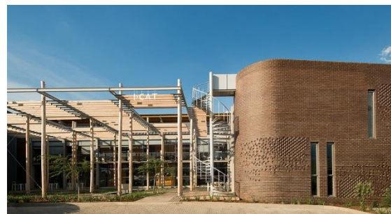
Figure 39: I-CAT factory, completed 2015 (Earthworld Architects, 2024: online).
