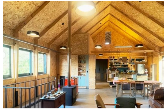
Figure 23: Use of plywood portal system at Plywood House, completed 2023 (Earthworld Architects, 2024: online).
