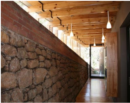
Figure 14: Juxtapose between stereotomic stone wall and tectonic timber frame at Gabriel's Garden (Kate Otten Architects, 2024:online).
