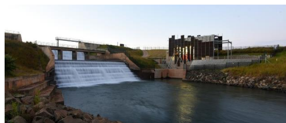
Figure 30: Stortemelk Hydro power plant, completed 2016 (Earthworld Architects, 2024: online)
