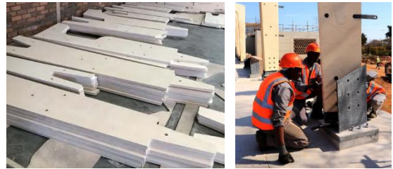
Figure 32: Hand assembly of CNC-cut plywood at Future Africa Campus, 2018 (Earthworld Architects, 2024: online).
