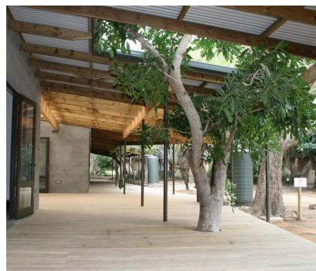
Figure 8: The roof is built around the existing tree at the WITS Rural Facility, 2016 (Kate Otten Architects, 2024:online).
