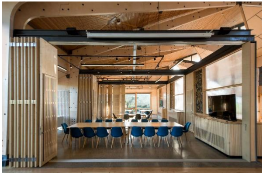
Figure 22: Use of plywood portal system at Future Africa Campus, completed 2018 (Earthworld Architects, 2024: online).
