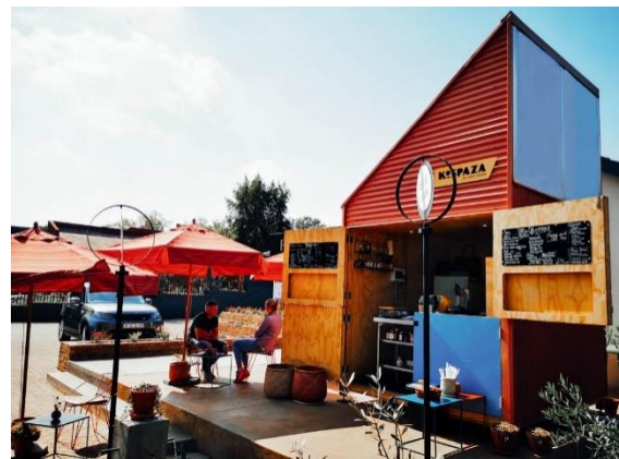
Figure 31: The KoSpaza Shop, completed 2021. (Earthworld Architects, 2024: online).
