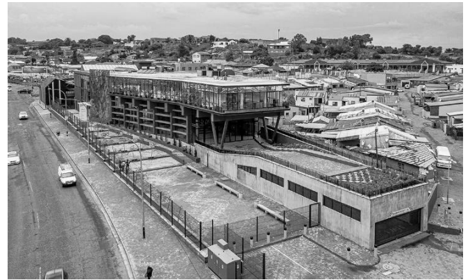
Figure 18: Fenced public space at the Westbury Transformation & Development Centre in Johannesburg (Takgalang Consulting n.d.).
