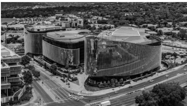
Figure 30: Discovery Place Sandton, Johannesburg by Boogertman + Partners showing stark contrasts with surroundings (Airgro n.d.).
