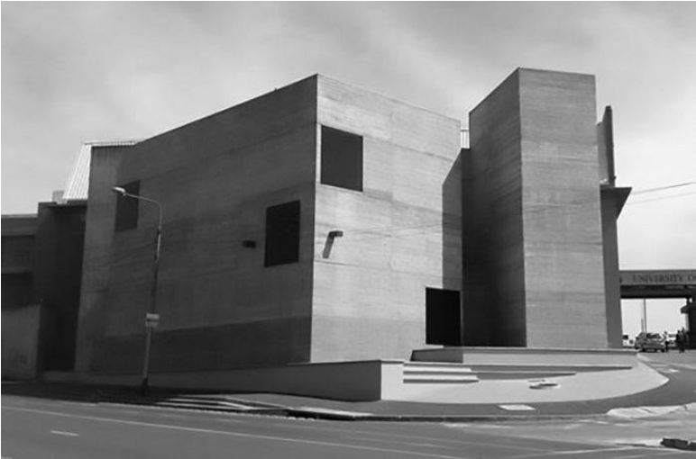
Figure 36: Origins Centre Rock Art Gallery, Johannesburg by Mashabane Rose Associates containing a secluded and inactive relationship with the street (Sherrat 2017).
