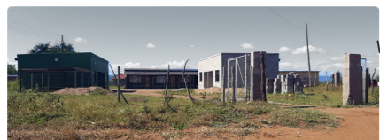
Lack of government support in residential property development
