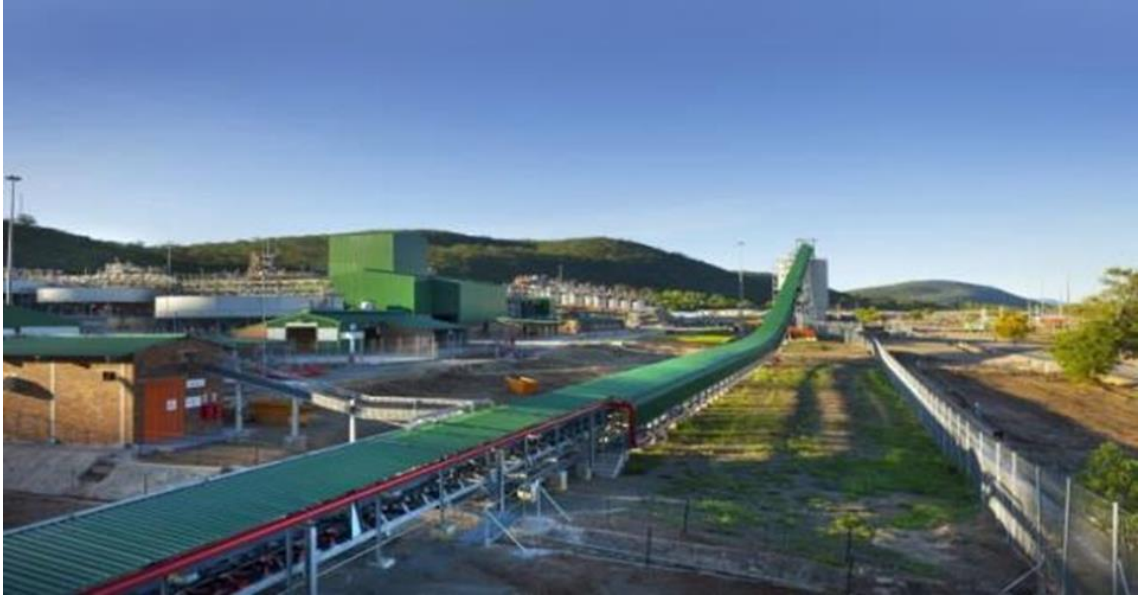
Figure 7.5 Unki mine plant (Source: https://www.angloamerican.com/ )
