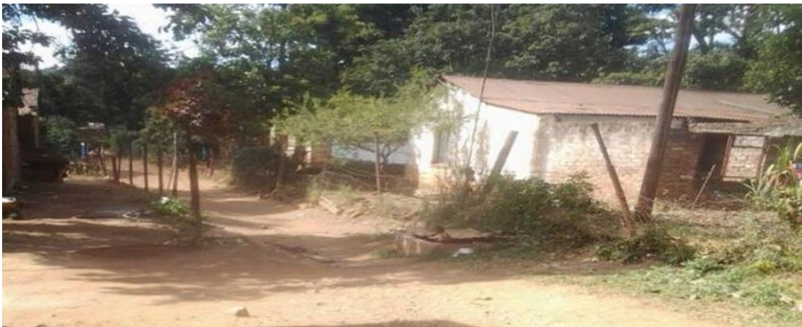
Figure 7.8 Dilapidated houses and roads in Makusha, Shurugwi Township
