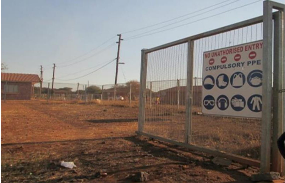
Figure 6.51 Entrance to the recently built family houses in Northam Extension 6. The compulsory PPE sign is still hanging on the main gate
