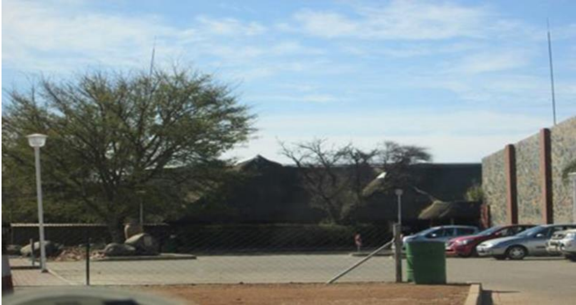
Figure 6.46 Multi-facility sports club that includes a tennis courts, gym, golf course and a swimming pool
