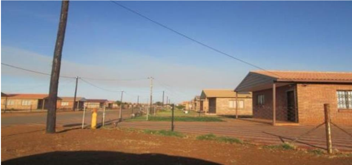
Figure 6.54 Neat rows of houses with electricity installed and tarred roads in good condition
