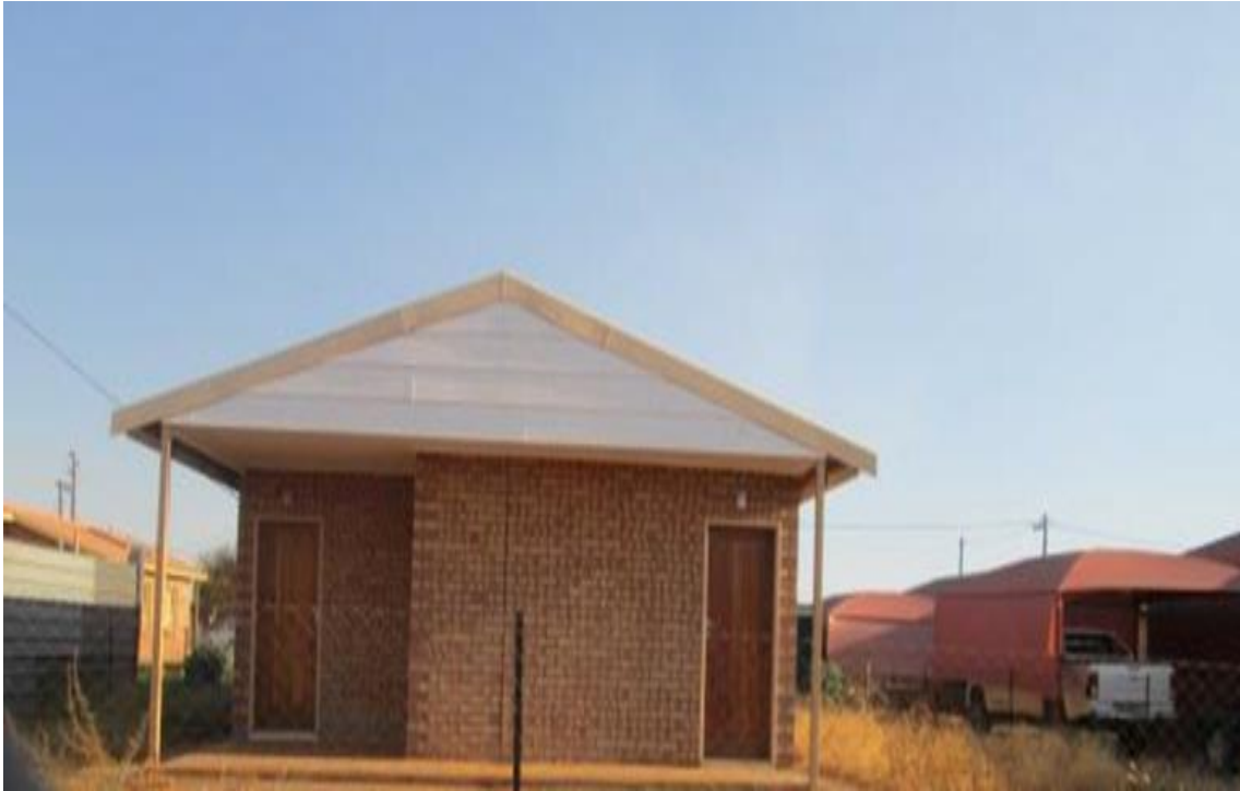
Figure 6.53 Unoccupied house at Northam Extension 6
