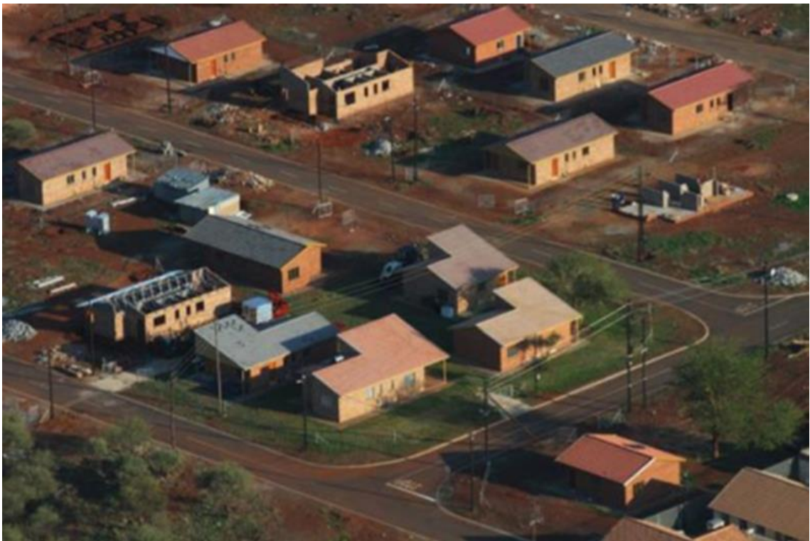
Figure 6.52 Aerial view of the Northam houses under construction
