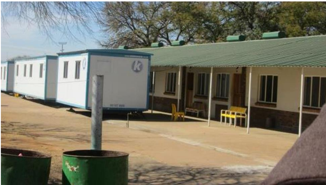
Figure 6.14 Tumela's containers for extra accommodation
