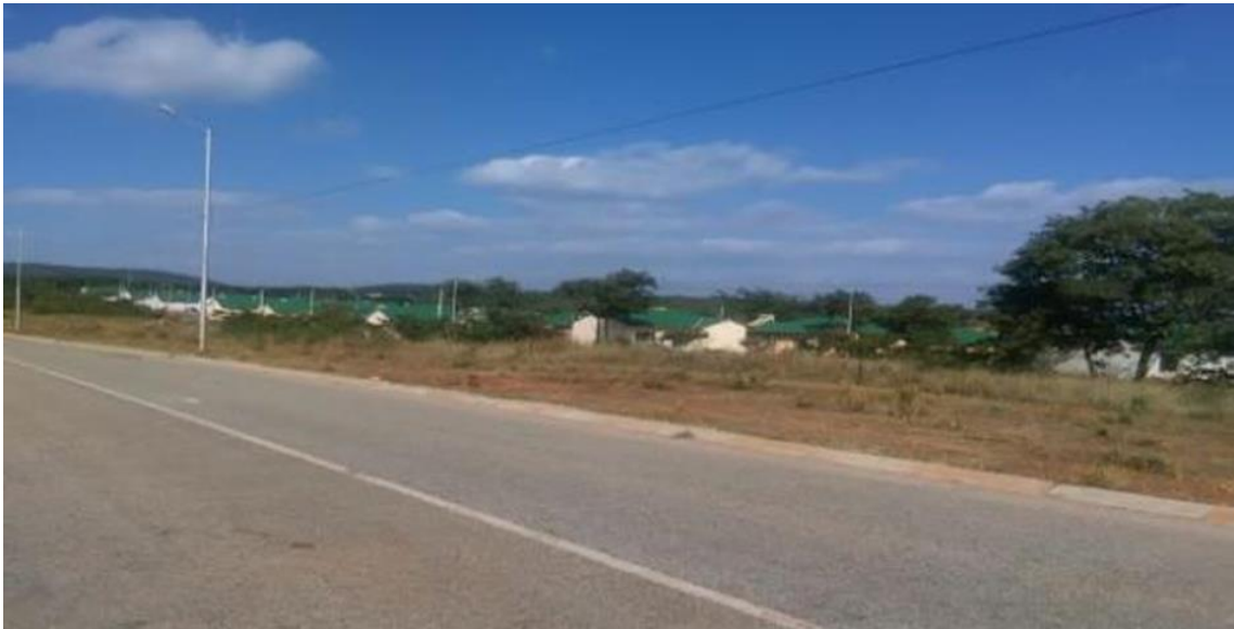
Figure 7.21 Detached spacious houses for shift bosses and artisans surrounded by natural vegetation
