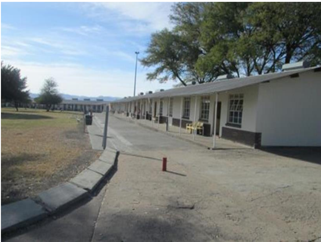
Figure 6.12 Mlanje SAV exterior view
