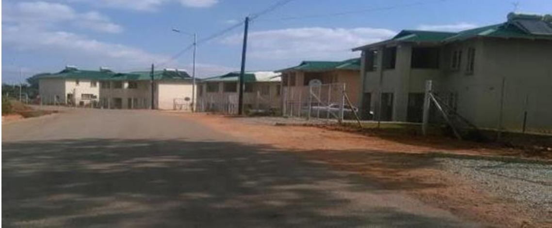
Figure 7.22 Three bedroom duplexes for entry-level underground mineworkers and their families
