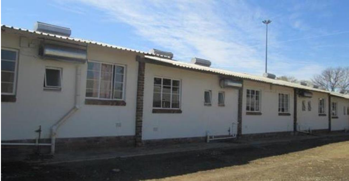
Figure 6.13 Each flat has a geyser installed for hot water
