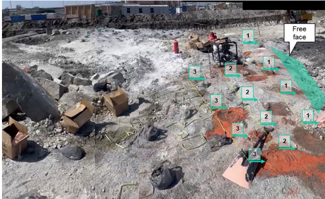
Figure 14—45 m diameter block being filled with the chemical
